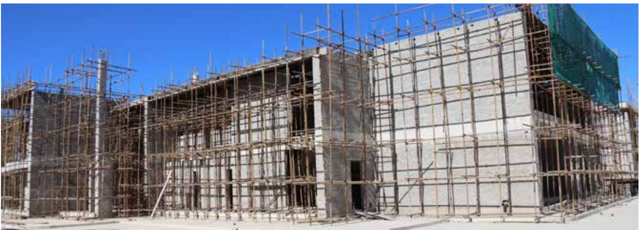
Ongoing construction of the new FIA Office Building
